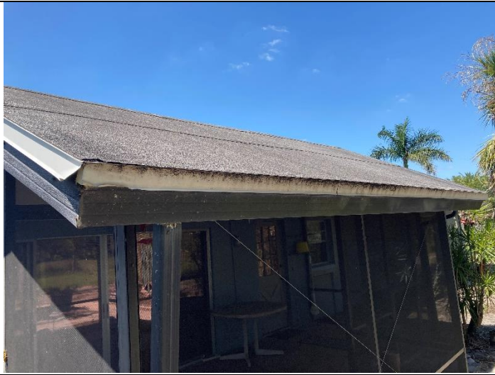
Photo 21: 7780 HA U - Rolled Asphalt Roof
